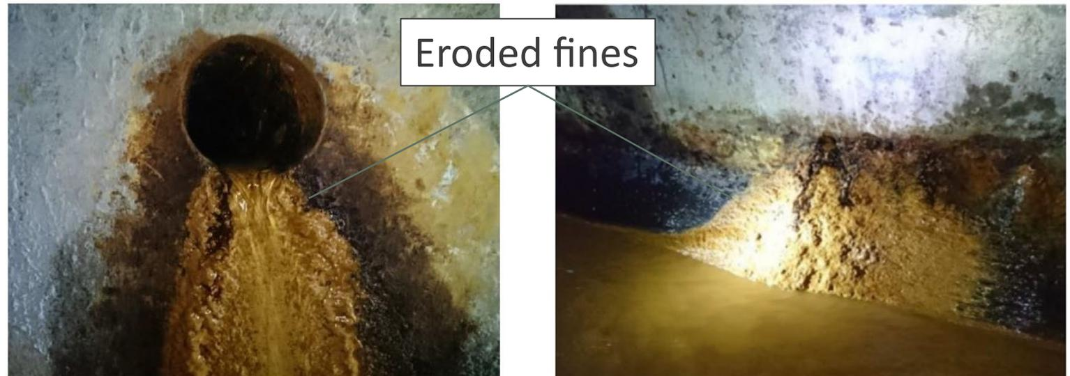
Picture 1: Layers of muddy cake inside underground drainage pipes.
